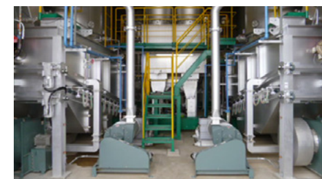
Biomass boiler, Nipro Pharma Odate Plant
