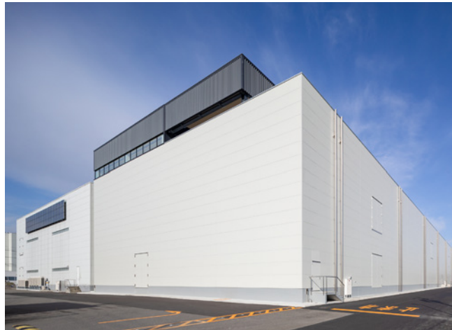
New building for pre-fillable syringe line under construction
