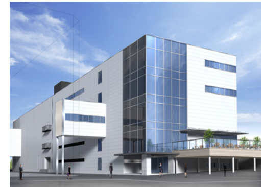
Image of a test area in the new building
