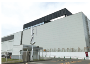
New building for pre-filled syringe line under construction
