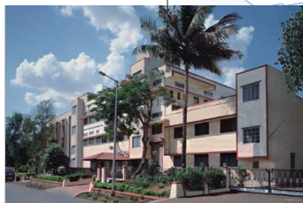
Nipro Tube Glass Limited Badlapur Plant
